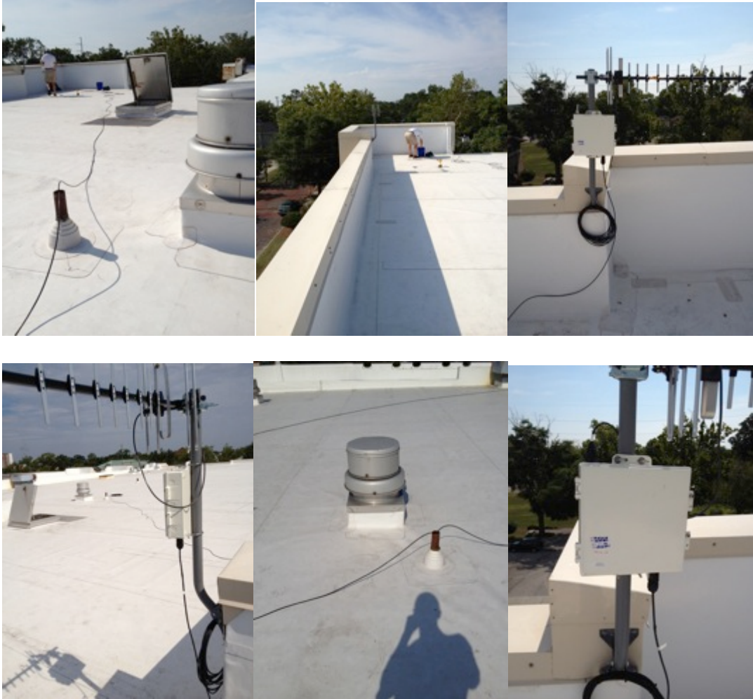
Figure 23: Cape Fear Museum Roof (source: William Edwards, 2012)
